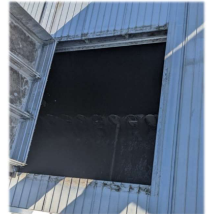
Figure 4. Primary Effluent Sampling Location
