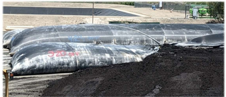
Figure 8. Dewatering Bags Sampling Location
